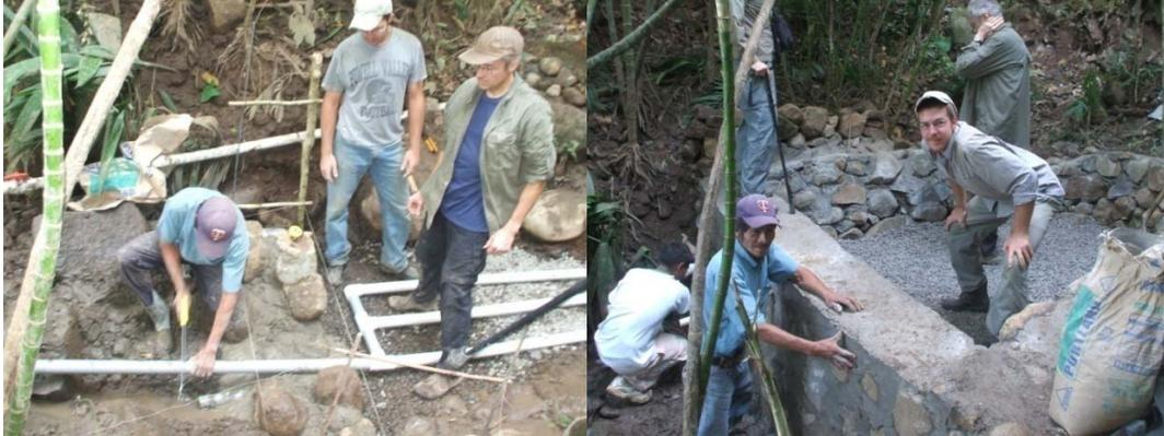
Figure 1: Left - Collection Screens in the bottom of the infiltration gallery. Right – Mason Don Maximino and PCV Jefferson Tyler Francisco in the finished infiltration gallery.
