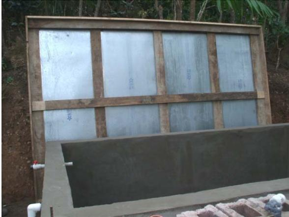
Figure 4: Underside of finished roof and finished plastered tank.
