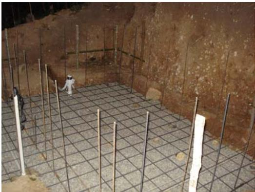
Figure 3: Rebar grid with vertical ties and drain piping.
