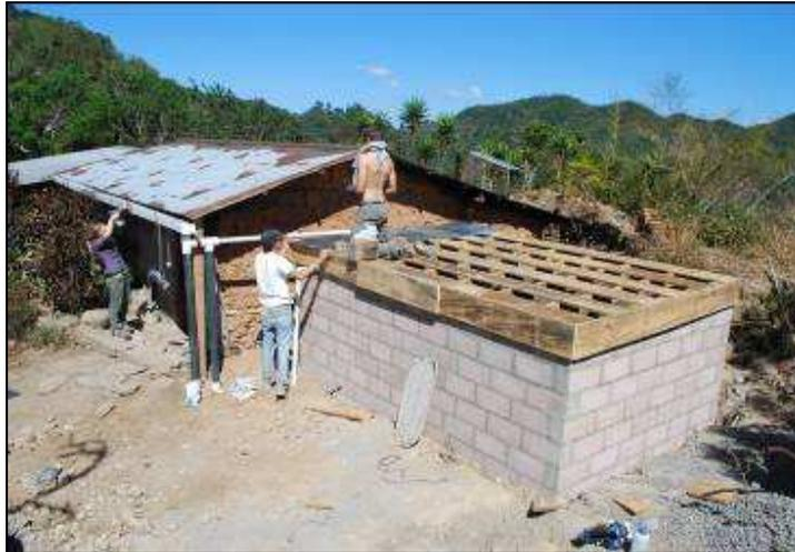
*Figure 3.3: Don Hugo's tank and partially completed roof. Gutters and first flush also shown.*
