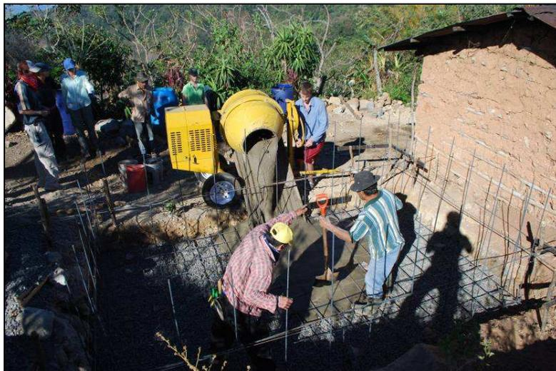
*Figure 3.1: Pouring the foundation of Don Hugo's tank with the cement mixer. The rebar grid can also be seen.*
