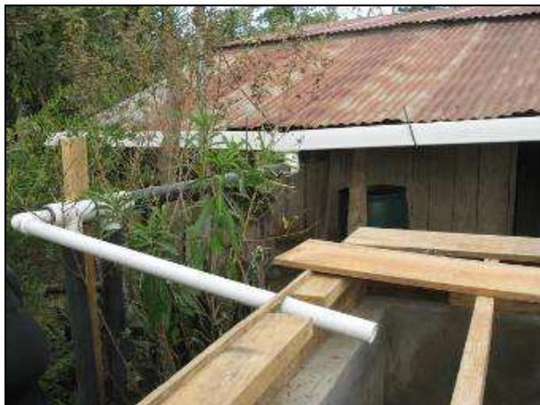
*Figure 3.2: Gutters, first flush, and inlet to tank at Don Jesus's house, prior to the tank roof being completed.*
