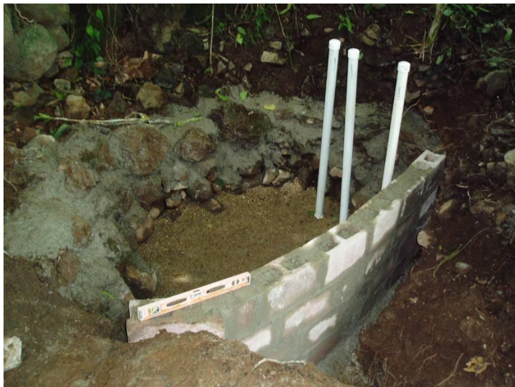
Figure 2.2.4 Infiltration gallery during the installation in December 2008
