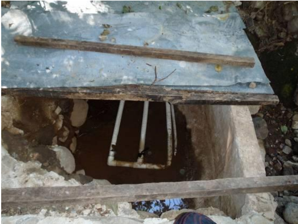
Figure 2.2.3 Excavated infiltration gallery in Las Mercedes
